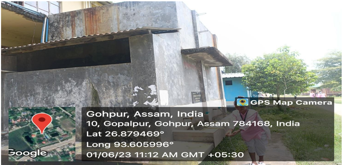
Water Storage Facility
