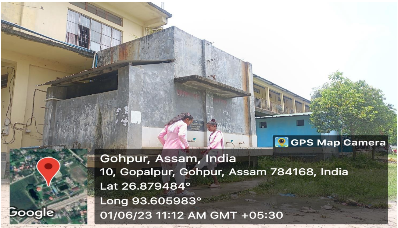
Water Storage Facility
